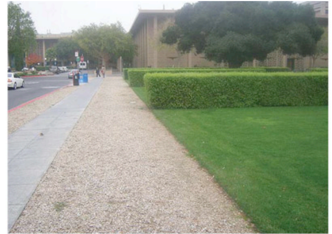
Compacted Gravel Paving
