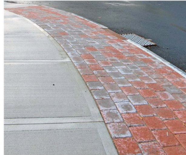
Concrete and Decorative Band at Edge of Asphalt
