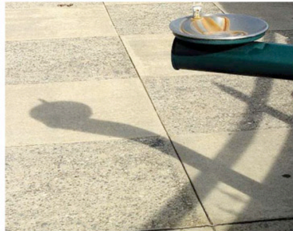
Grey Concrete and Exposed Aggregate Concrete
