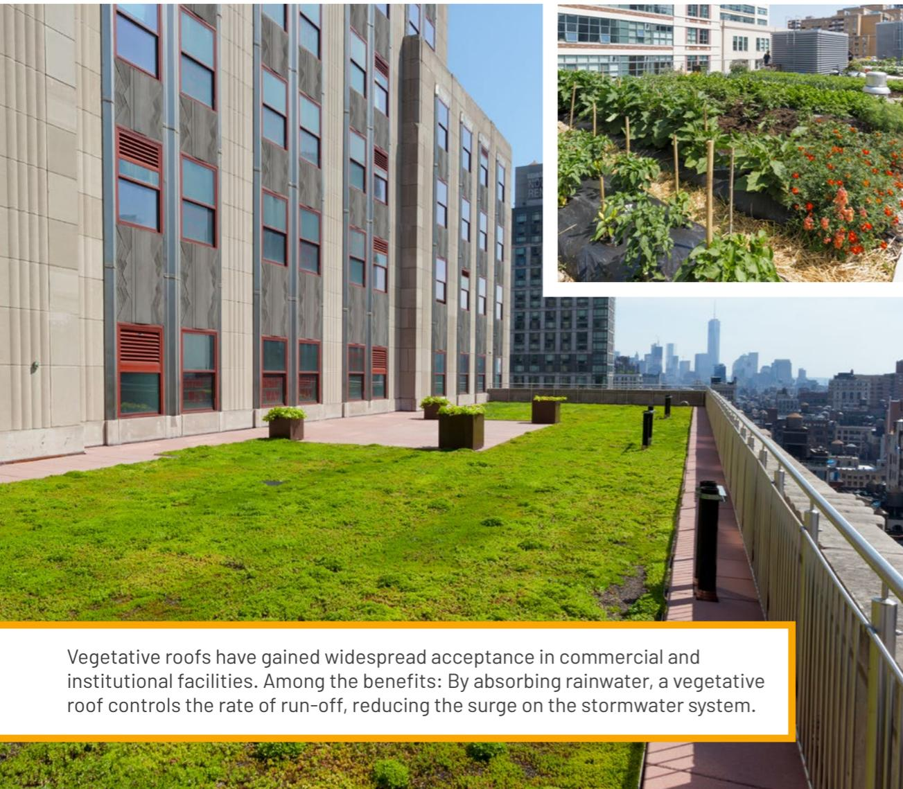
Vegetative roofs have gained widespread acceptance in commercial and institutional facilities. Among the benefits: By absorbing rainwater, a vegetative roof controls the rate of run-off, reducing the surge on the stormwater system.
