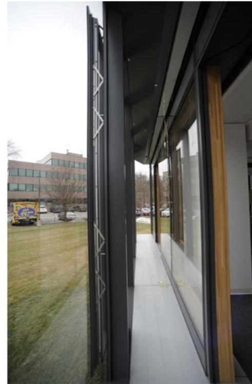
The Tower at PNC Plaza has a double-skin façade that was tested in a 1,200-square-foot-mockup. The 30-inch cavity between the double walls of the façade insulates against heat loss in winter and heat gain in summer. The exterior wall also features glass air gates that open to allow outside air to enter the cavity when conditions are right. (Inset photo shows a mockup of the double-skin façade.)
