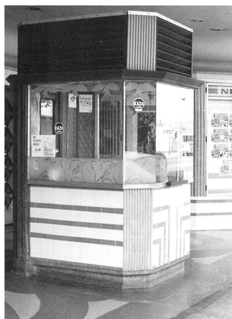
Garden Theatre entrance on Lincoln Avenue in San José's Willow Glen neighborhood, circa 1981. The one-time movie house has been reconstructed to accommodate retail businesses.
